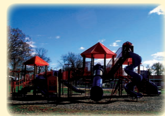
Peterson Park Playground
